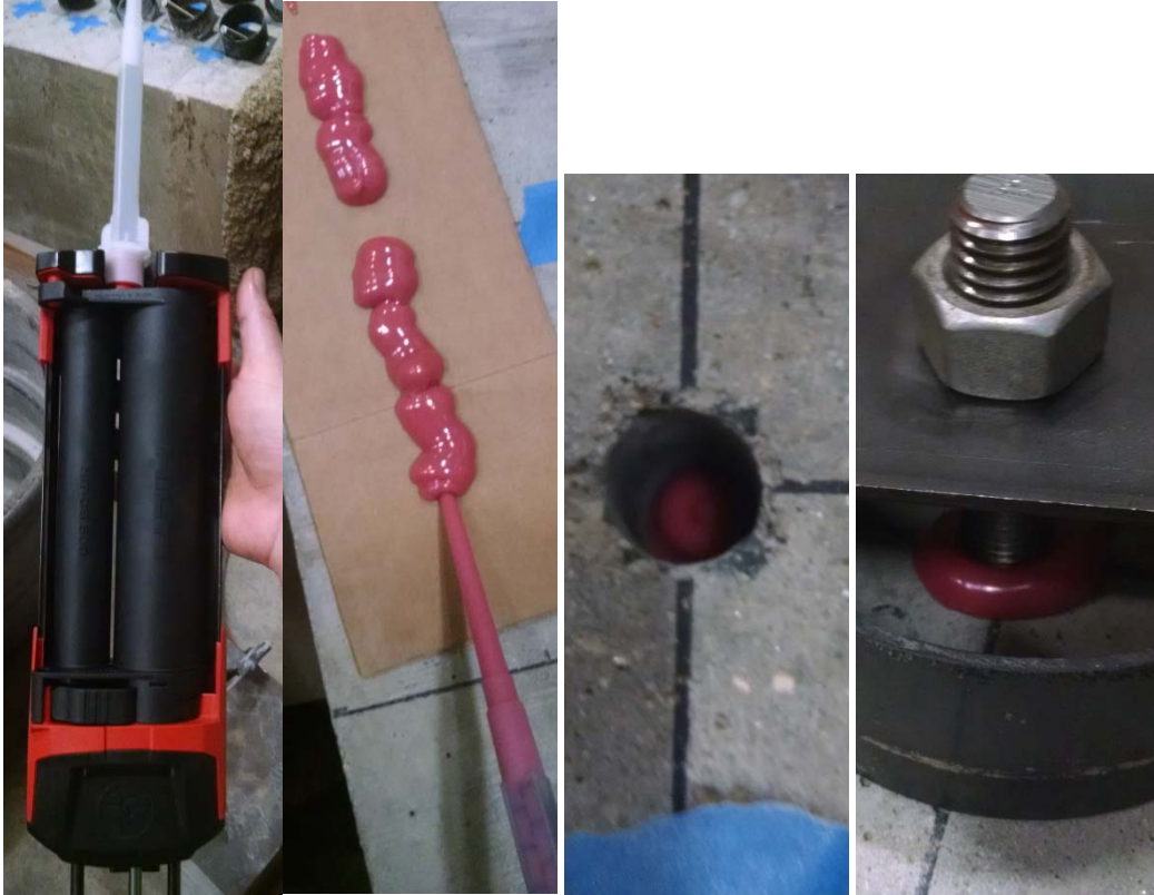
Figure 8.9 Adhesive Application
