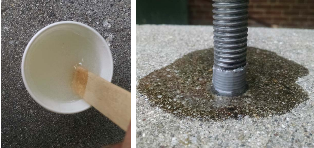
Figure 8.4 Mixed Epoxy (Left) and Installed Anchor (Right)
